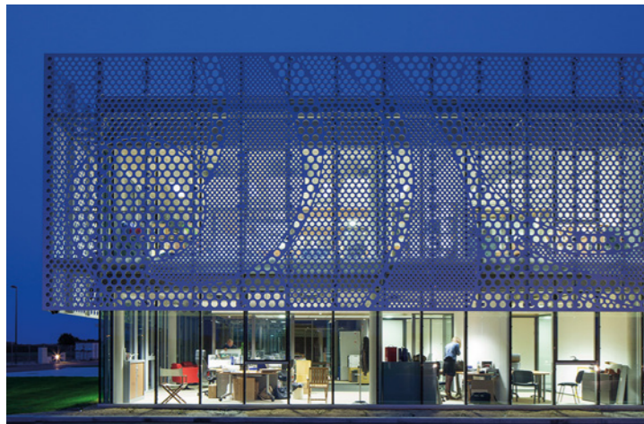
Design: PAD Architectes for BERI 21 | Fabrication: LCCA | Photo: Mathieu Ducros
